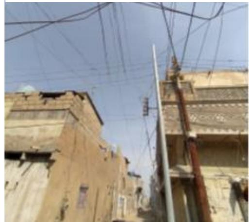
A major component of the project was upgrading supply lines at the Pole Mounted Transformer (PMT) level to Aerial Bundle Cabling (ABCs). Due to their intertwined cable design, ABCs are difficult to connect to using "kundas", making it physically harder to attach illegal lines to them. While ABC conversion pre-dates the project, it was a major component and also the most visible aspect of the project, and we therefore analyse its effects separately as well.
